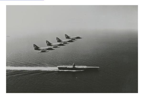
A 1962 photograph of A-4D-2N Skyhawks from VA- 76 fly over *Enterprise* with hooks down in preparation for their approaches and arrested recovery. The *Big E* is steaming into wind at speed, with almost a rooster tail in her wake! (USN photo)
