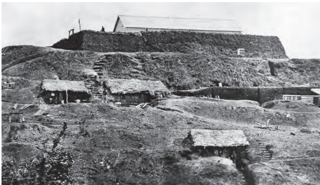
The Pihiri Redoubt, circa 1866, defines a well built and defended strongpoint. The Military Settlers accommodation was outside of the Redoubt and built into the ground. The redoubt was on a high point with the advantage of a long field of vision.
